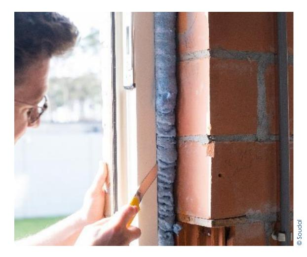
After application, these products are always covered by, for example, doorframes, window frames or plaster. They are used exclusively on the inner shell of buildings, and contact with the outside environment will not take place. Excess foam will be removed by cutting it with a sharp knife after the foam has cured, so no contact with the polymeric precursor takes place.
