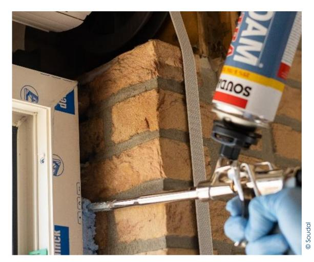
Application by a professional worker of OCF, containing the polyurethane precursor, in a window frame
