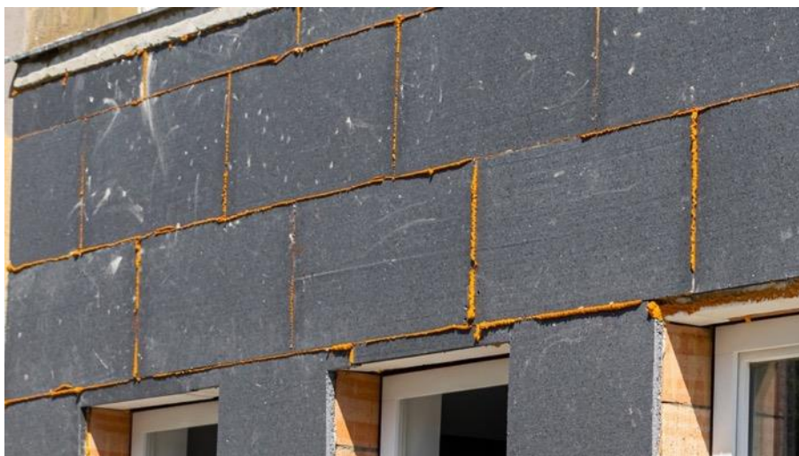
Figure 5: Use of polyurethane foam to fill gaps in external thermal insulation systems.
