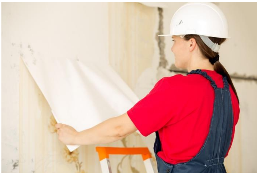
Figure 19: Mechanical removal of old wallpapers can include selective release to leave a clean surface.
