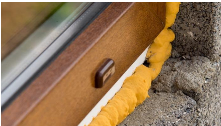
Figure 4: Use of polyurethane (PU) foam for insulating gap filling around window elements.
