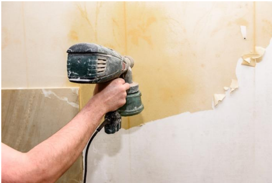
Figure 20: Soaking of wallpapers for easier removal, a form of debonding.
