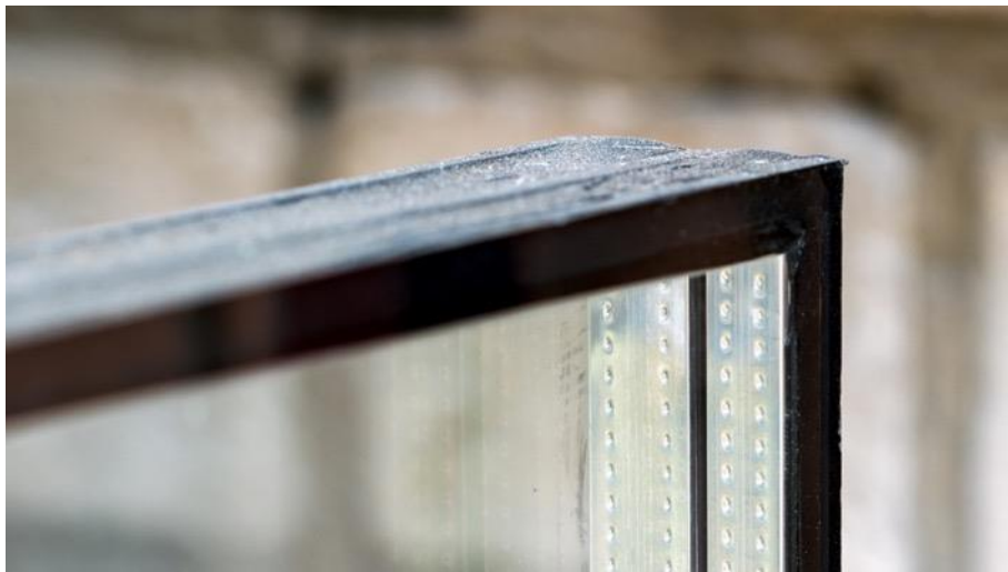
Figure 9: Closeup of the sealed edge of a multipaned glazing element.
