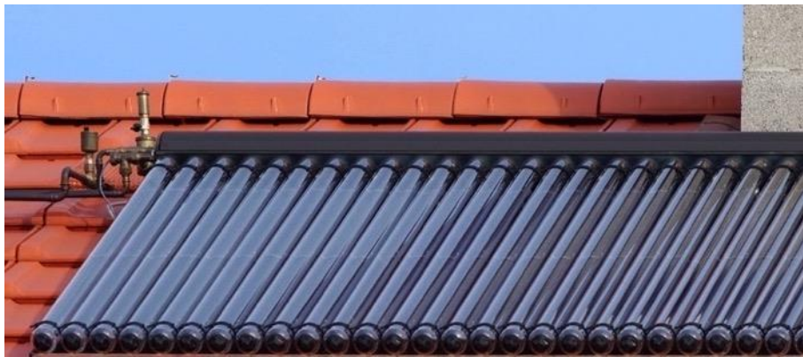
Figure 12: Solar thermal units can replace conventional warm water heaters.
