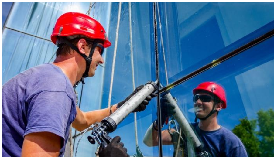
Figure 16: Maintenance of a glazed window front with a façade sealant.
