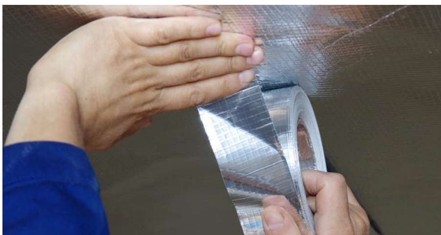
Figure 6: Use of self-adhesive tape to provide airtightness along the seams between in-roof insulation panels.
