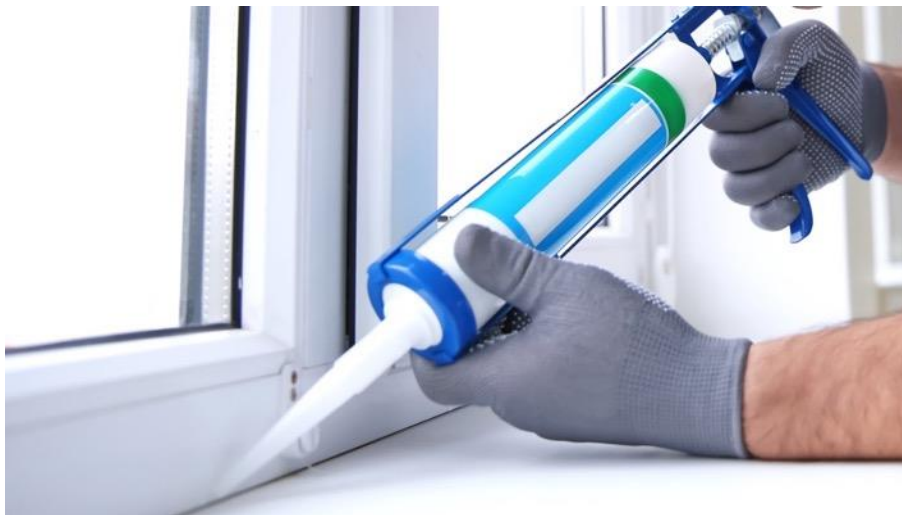
Figure 7: Use of silicone sealant to provide airtightness around a window frame.
