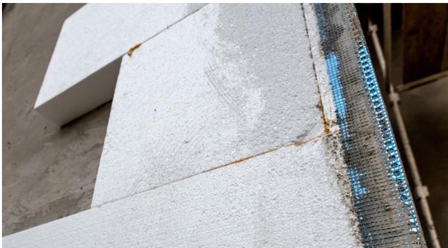
Figure 3: Installation of an external thermal insulation system with adhesives instead of mechanical anchors.
