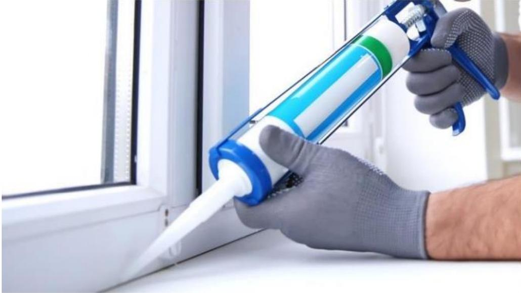
Sealants are used to seal cracks or joints and serve an important role in building and home design.
