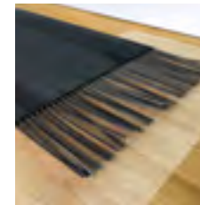
Prepare the belt to be jointed (Arrange the exposed steel cords)
