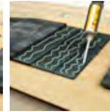
Add the adhesive using an application gun
