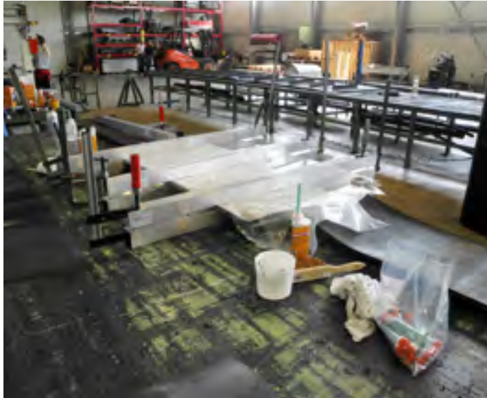
Bonding of conveyor belts in the workshop.
