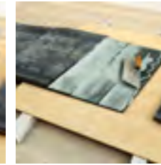
Evenly distribute the material to roughly 1 mm thickness
