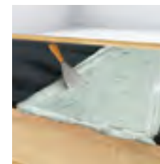
All steel cords have to be well embedded within the adhesive
